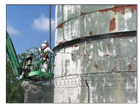
CTI first needed to make sure the crew could work as safely and efficiently as possible. CTI utilized two 60' JLG Lifts to access, prepare, and coat the Surge Tank, utilizing their certified and experienced operators.
