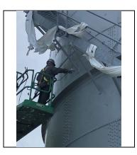
← Applying Coating from JLG Lift Basket utilizing Sprayer
