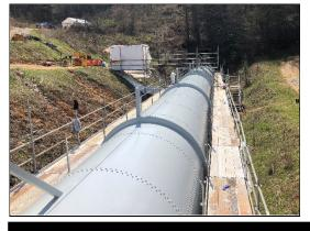
The CTI team coated the Penstock with a 3 Coat System that will provide UV and Corrosion protection to withstand the extreme environmental conditions.
