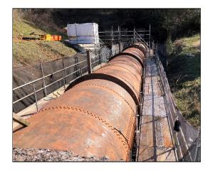
Prior to preforming the coating CTI needed to ensure a clean and smooth surface. For this particular project CTI utilized ROTO Pen DECO Tool and Needle Guns on a 11' Diameter Penstock Pipeline to produce a SSPC 2/3 Surface Profile.
