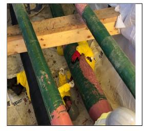
The pipes were then prepared for wrapping activities through putty application, smooth transitions, surface cleanliness, and surface irregularities that were then checked and approved by one of our experienced NACE III inspectors.
