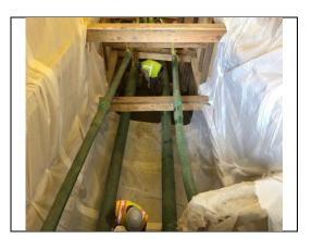
Prior to any application, the work area is prepared to accommodate the installation of the Carbon Fiber Wrap System; which includes installing FR Sheathing for proper environmental protection around trench area.
