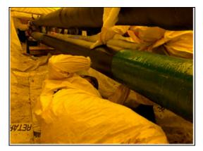
After these steps, our 6 Layer Carbon Fiber Wrap System consisting of properly mixed components, properly saturated fabric, and applicators applying saturated product onto pipe under correct supervision and controlled environmental conditions.
