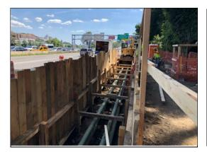
CTI specializes in applying effective reinforcement systems that help strengthen rather than replacing the structure itself. For this customer CTI applied a carbon fiber repair system (6 layers) and three coats of topcoat to protect the exterior of four buried oil/electrical pipes (5" and 10") from erosion.
