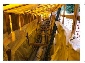
After the Carbon Fiber Wrap System is applied the surface area is inspected for Voids, Air Pockets, Lifted Edges, or any other irregularities by NACE III inspectors. If any irregularities are found they are marked, removed, and repaired.
